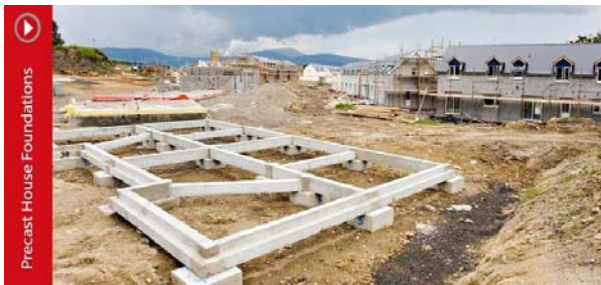
Figure 1. Precast foundations Source: http://terradrive.ie/wp-content/uploads/2014/04/accordion_house.jpg
